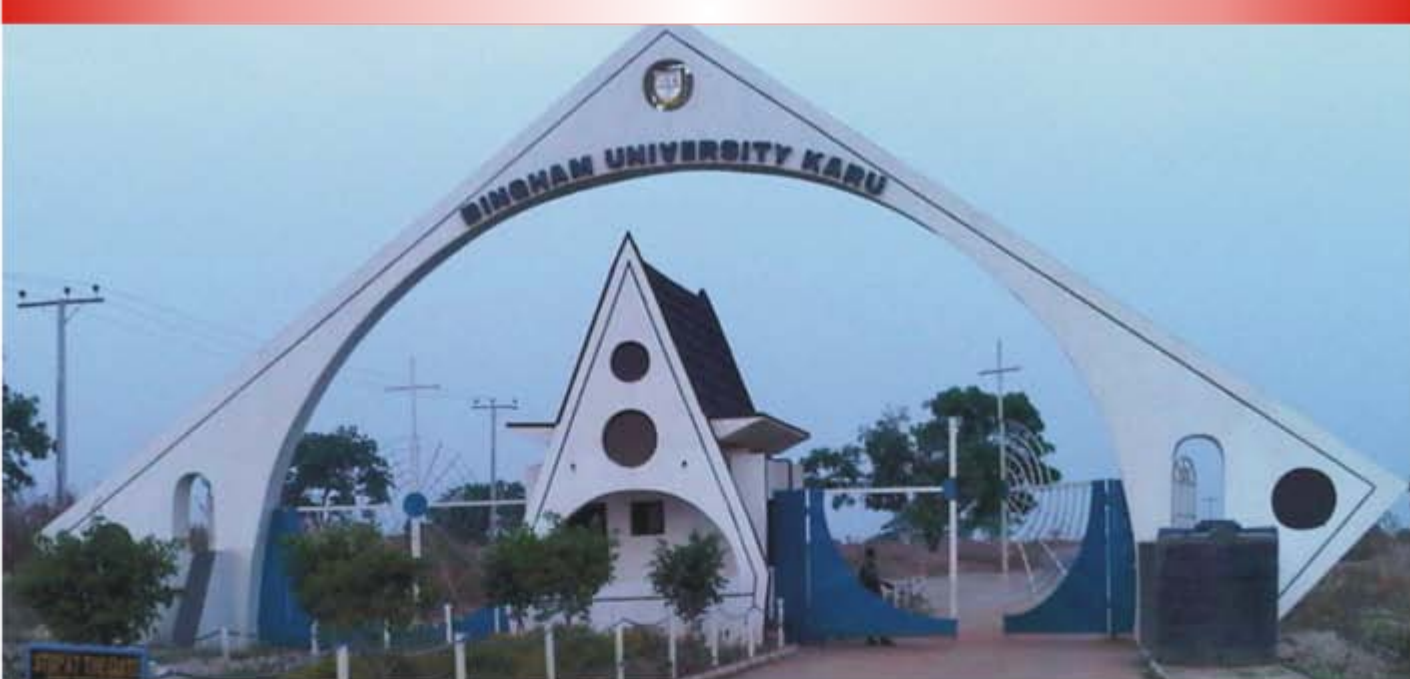
Main Entrance Gate of the Bingham University, Karu
